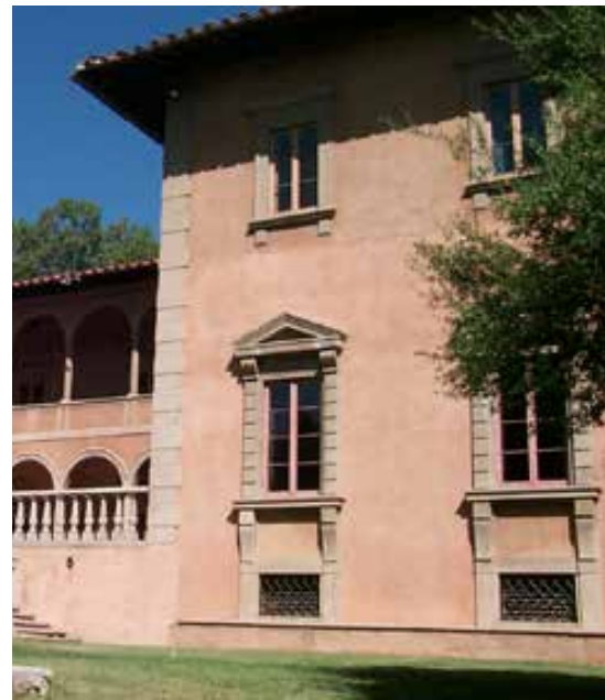
Smooth Trowelled Plaster
