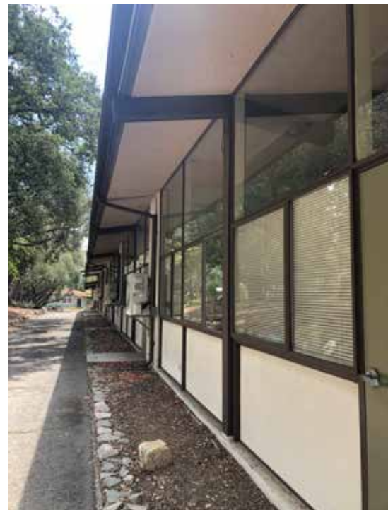
Exposed wood structure, deep overhangs, and clerestory windows will connect the new buildings to existing mid-century architecture
