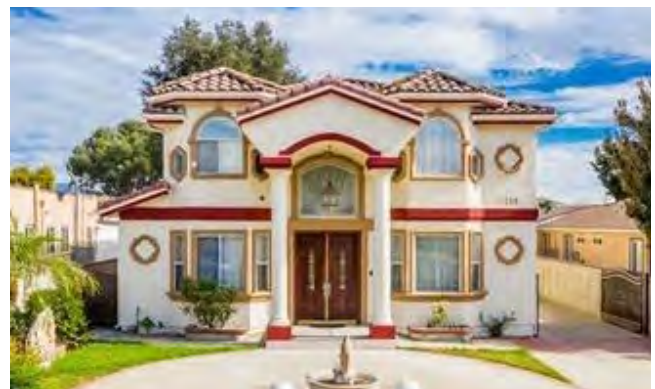
Inappropriate: Oversized, monumental primary door entry elements, e.g., two-story columns.
