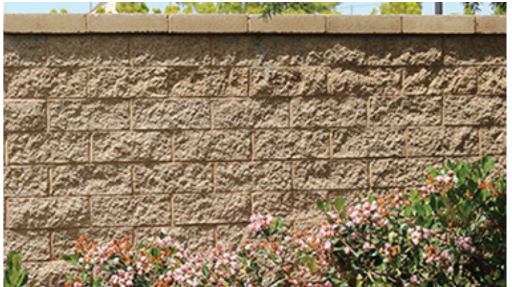
— Retaining Wall (Height Varies)
