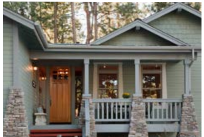
Appropriate: Primary door entry is visible, identifiable, and emphasized by use of a porch.
